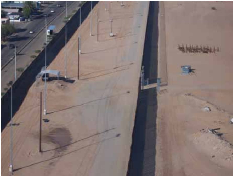
Double-layer fencing plus surveillance technology.
