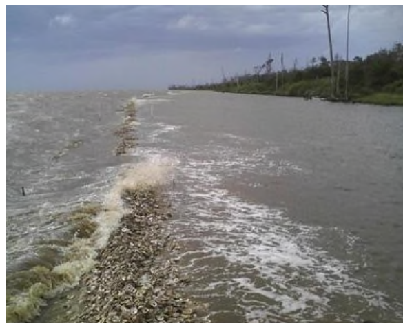
Figure 4-3. Installed oyster breakwaters at Bon Secour Bay, AL.
